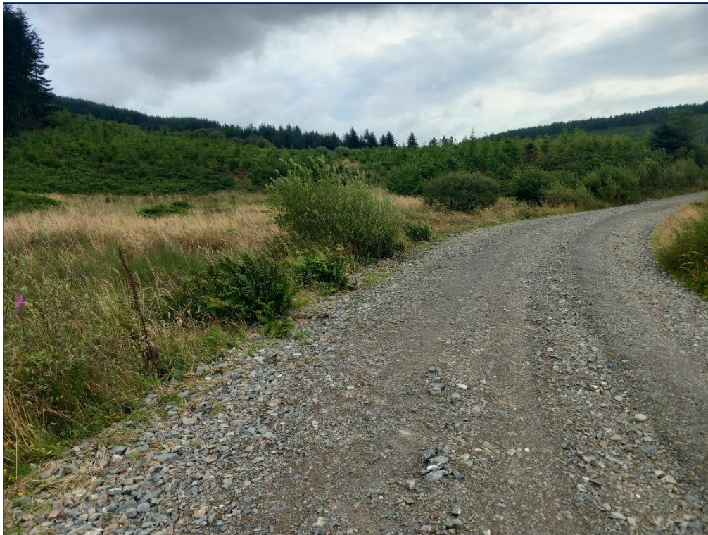
Plate 10-46: East facing view of the Access Track from the western extent of Glengap Forest
