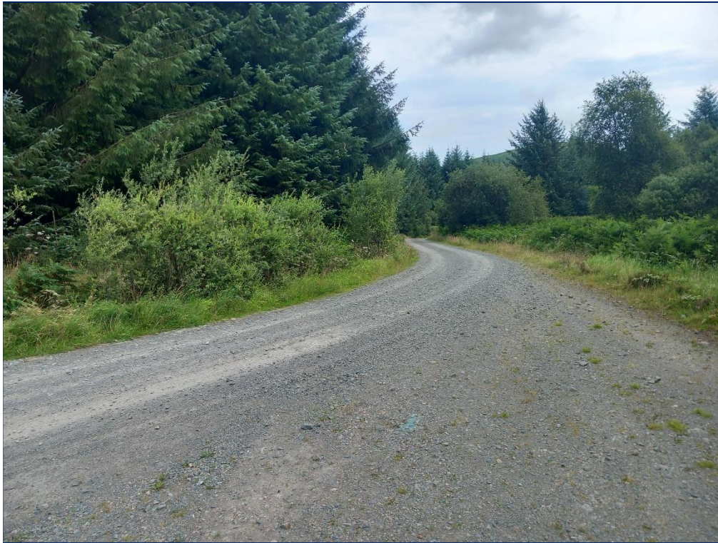
Plate 10-48: East facing view of the Access Track, west of Glengap
